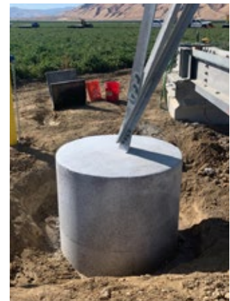
Fig. 21 & 22: New foundation poured and finalized
