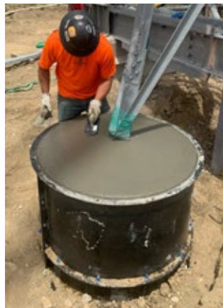
Fig. 21 & 22: New foundation poured and finalized
