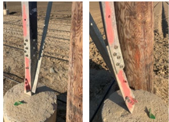
Fig. 2 & Fig. 3: Tower M36-T2 leg damage
