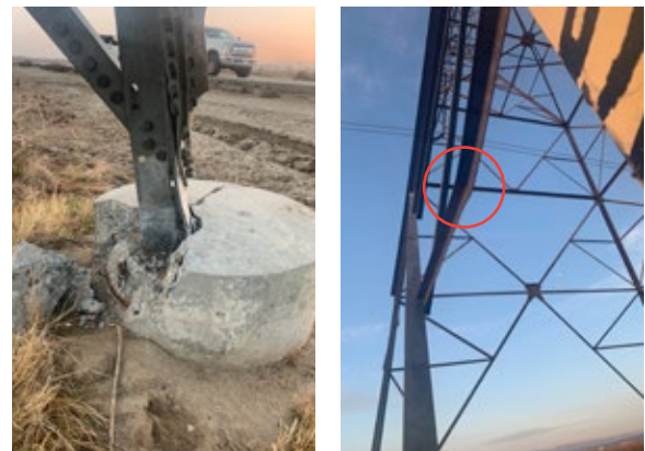
Fig. 4 & Fig. 5: Tower M15-T3 foundation and lattice tower damage
