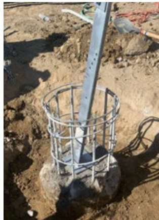
Fig. 19 & 20: Repaired leg ready for new foundation
