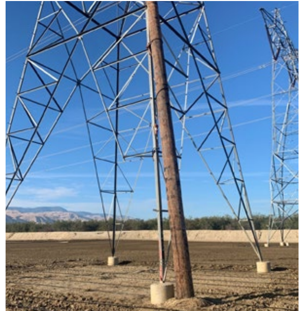
Fig. 1: Tower M36-T2 leg held up with wooden pole
