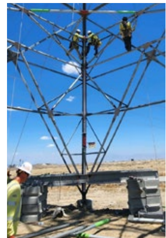
Fig. 15 & 16: Finished foundation upgrades enabling tower work
