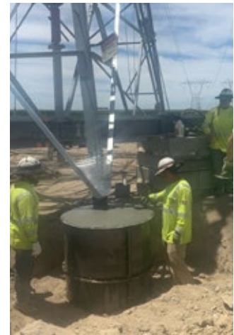
Fig. 13 & 14: New foundation concrete being poured
