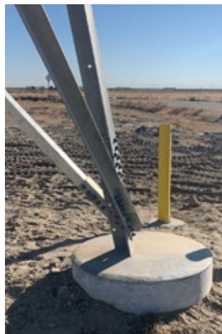
Fig. 15 & 16: Finished foundation upgrades enabling tower work
