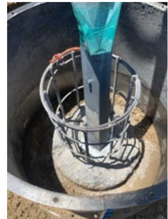
Fig. 19 & 20: Repaired leg ready for new foundation
