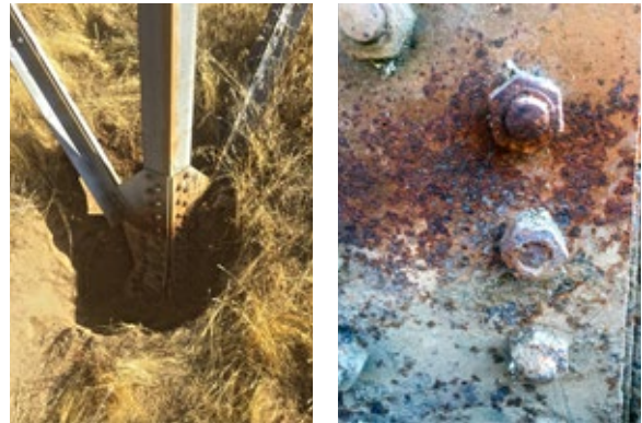
Fig. 2: Corrosion damage
