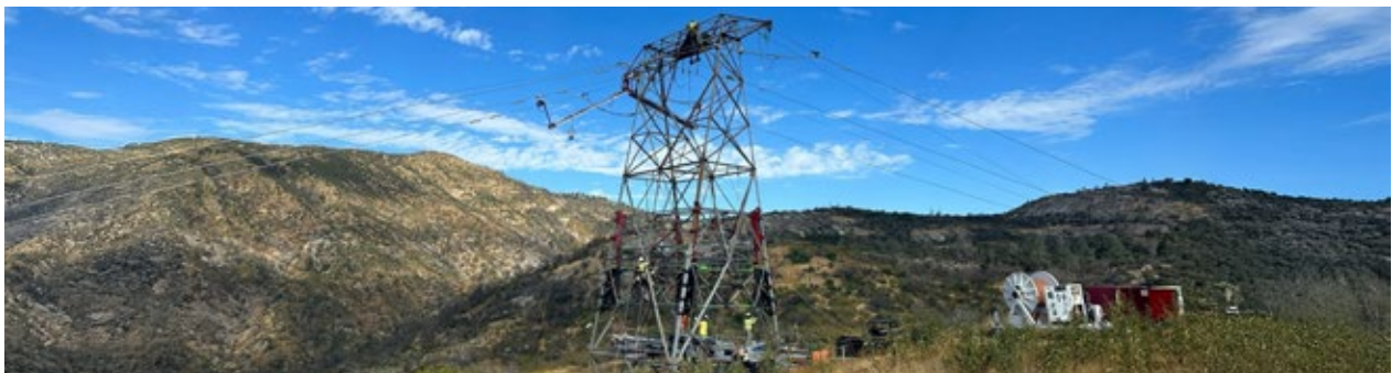
Fig. 9: Crew safely performing tower raise using the Ampjack® system
