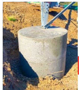
After corrosion repair
