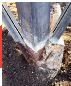
Before corrosion repair
