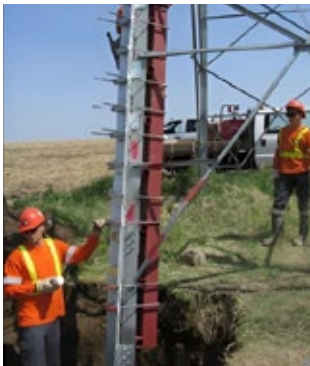
Leg repair during and after
