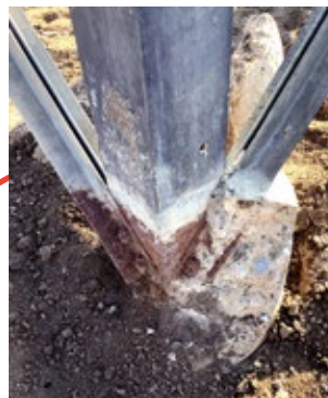
Before corrosion repair
